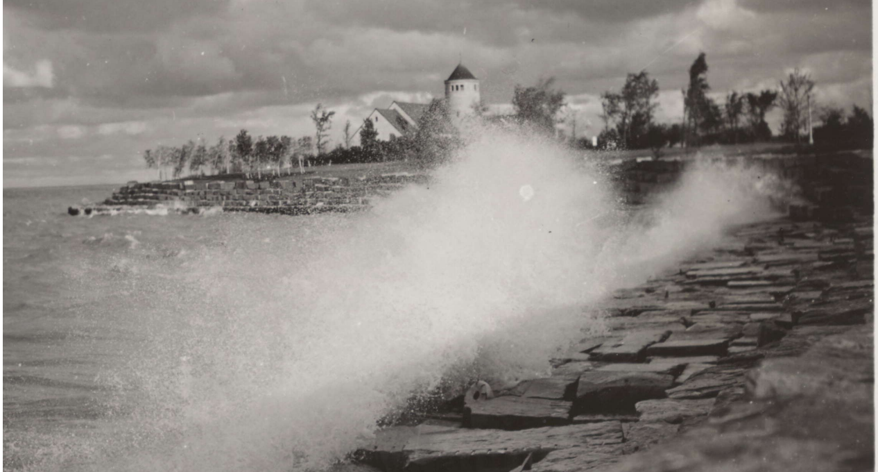
Above: Looking southeast across step-stone revetments toward pavilion, circa 1940. (Source: Chicago Park District Records: Photographs, Chicago Public Library Special Collections)
